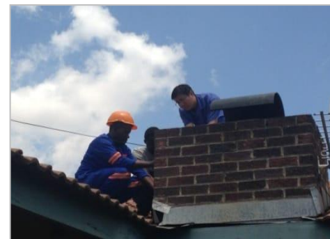
Fig-8 Drop Cable Installation
