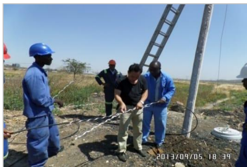
Cable Fittings Installation
