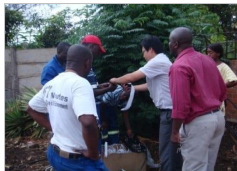
Closure/splitting box Installation
